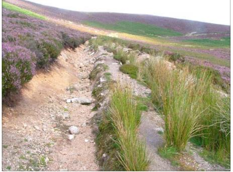
Poor construction of tracks without adequate drainage leads to serious erosion, Here, in a bulldozed track near Clach na Ben erosion has removed both sides of the track that would support vehicle wheels to a depth of about 30cm, leaving a narrow strip high in the middle.
