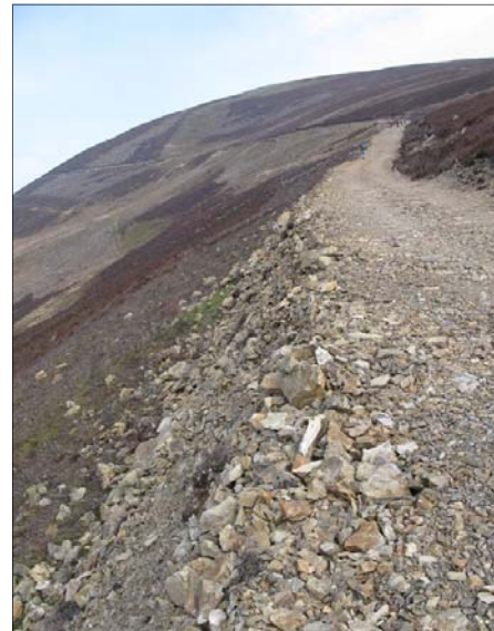
Massively engineered bulldozed track on Millden Estate in Glen Esk
